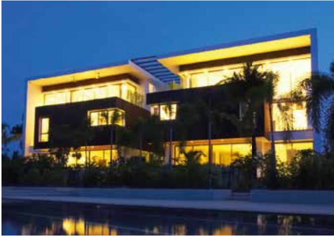
...for emergency power supply
